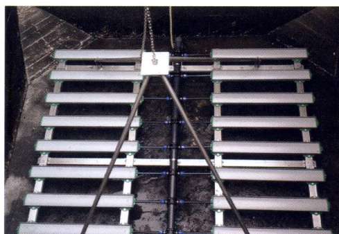
Collegamento tra due diffusori Connection between two diffusers
